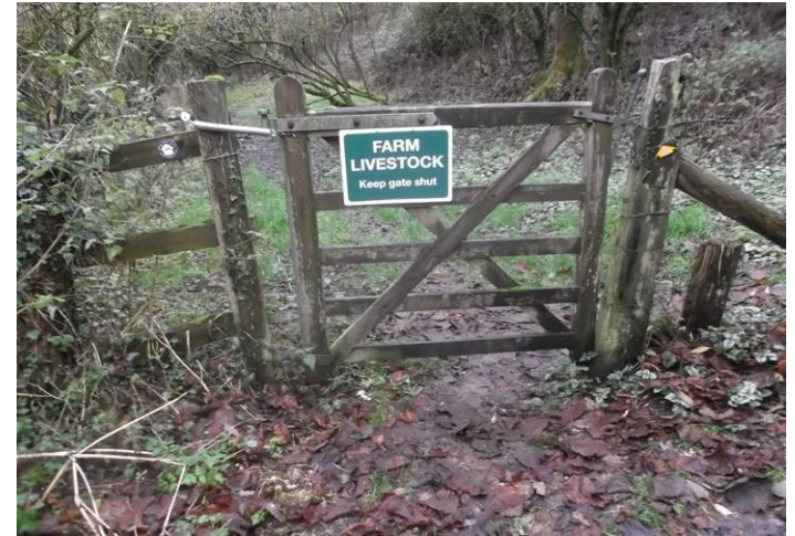
17. Looking east uphill. RH gatepost requires replacing or straightening.
